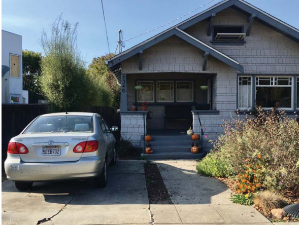
Figure 2: Existing parking space
